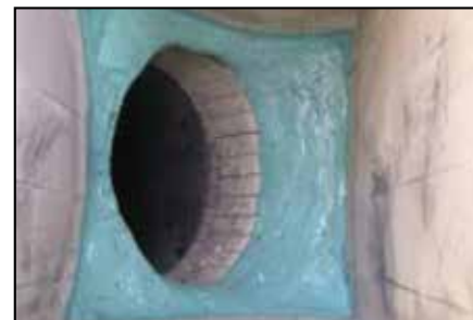
ARC BX5 with ARC S2 topcoat cures rapidly, allowing fast return to service of chute.
