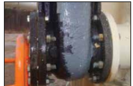
Repaired valve with ARC 5.
