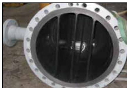
Repaired divider plates.
