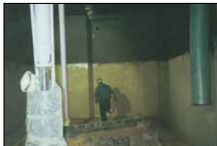
Concrete protected with ARC 791 and ARC 988 .
