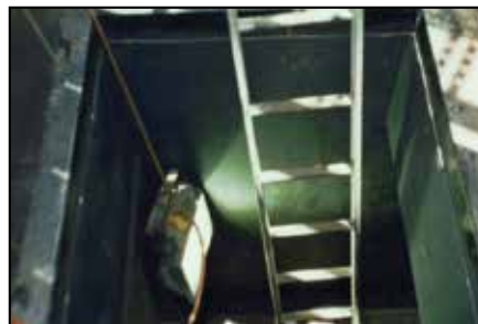
ARC specified by plant engineer.
