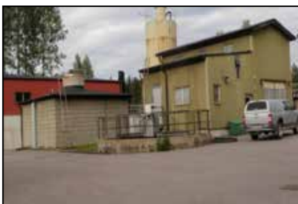
Wet well location.
