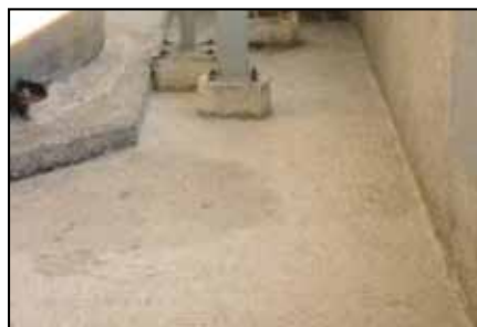
Cleaned and prepared surface.
