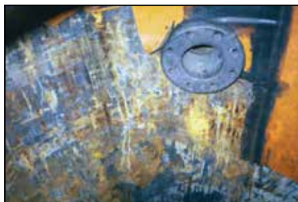
Removal of the rubber lining in progress. Blistering of the lining is visible.
