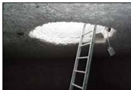
Surface of wet well high pressure cleaned and abrasive sweep sandblasted.
