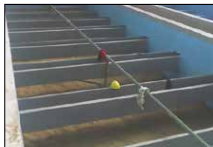
Installing ARC S1PW coating.
