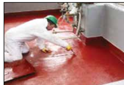
Applying ARC CS4 topcoat.
