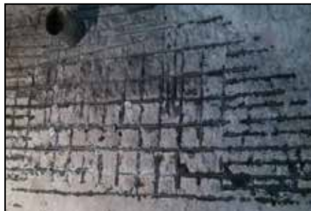
Chest wall after tile removed and blasted.
