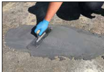
ARC EG-1 applied to concrete.
