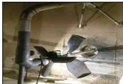
Mixer and lance with the applied ARC 855 and ARC BX2 coatings.
