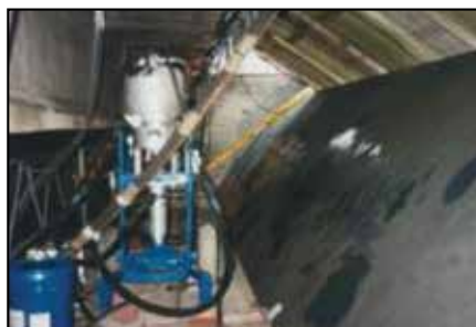
Pitting repaired using ARC 858 .
