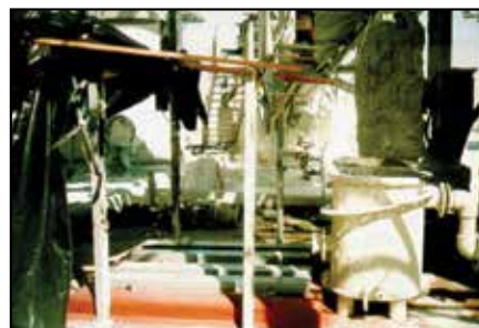
ARC 988 coated processing areas.
