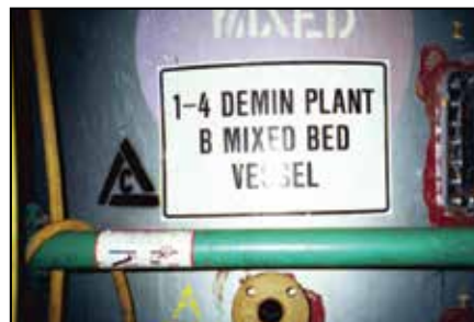
External view of the tank.
