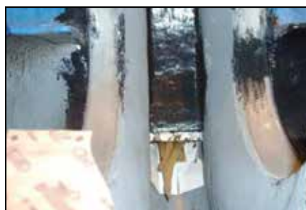
Pumps rebuilt with ARC 858 and ARC MX2 . Top-coated with ARC 855 .
