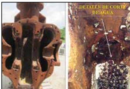
Pump body as inspected.
