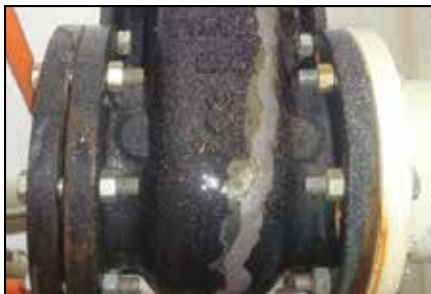
Valve leakage plugged with ARC 5ES.
