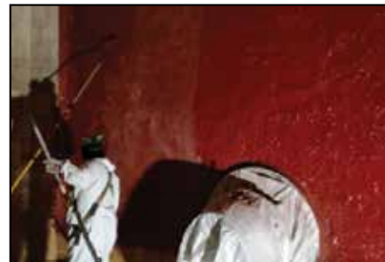
Applying ARC NVE sealer coat.
