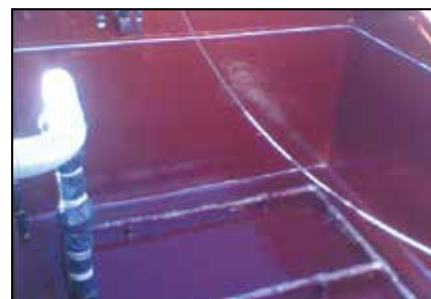
ARC CS4 final application.
