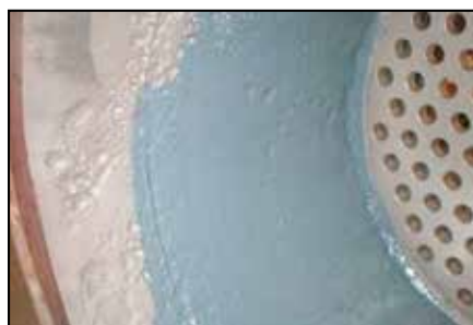
After application of ARC 858 , ARC SD4i is applied for protection and enhanced flow efficiency.
