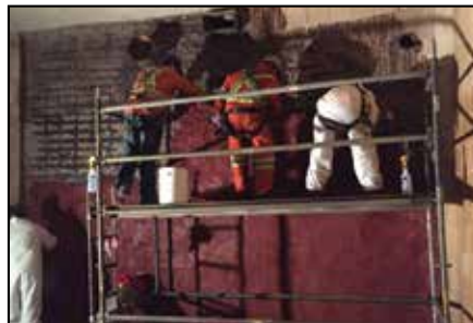
Installing ARC NVE coating.
