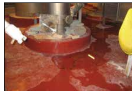
ARC NVE VC in service.
