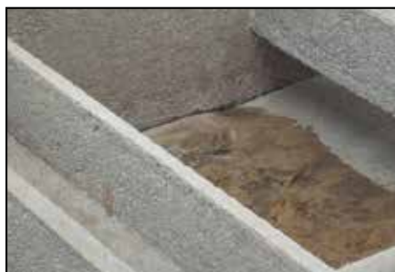
Drained sand filter vessel.
